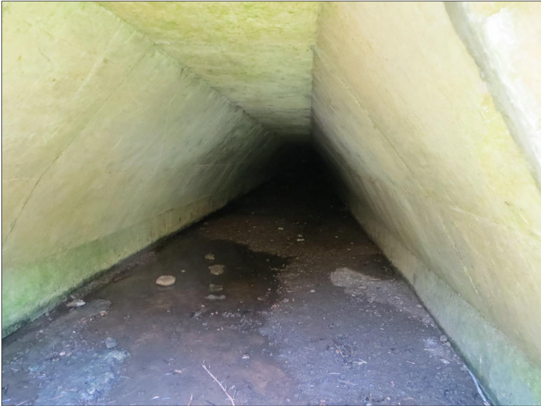
Figure 5.4 – Culvert under A508 Roundabout
