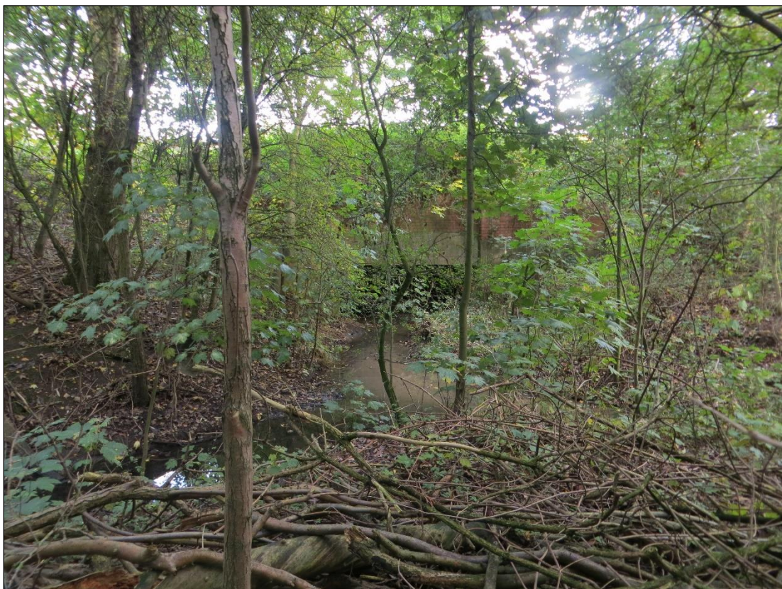
Figure 5.3 – Courteenhall Brook flowing into M1 Culvert
